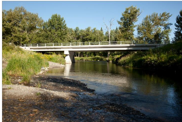
East Hillcrest Bridge – 2019
