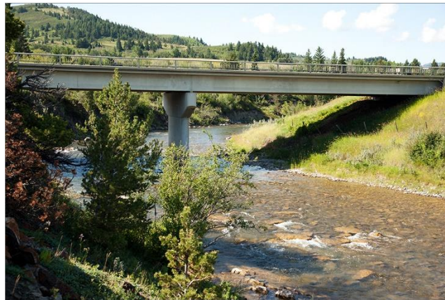
Hwy. 3 Bridge, Lundbreck – 2019
