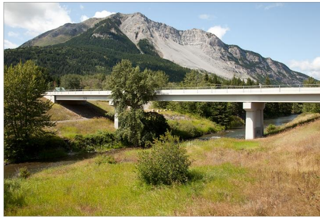
West Hillcrest Bridge – 2019
